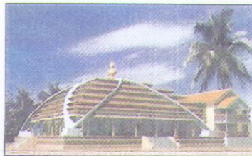
Perspective View of Gurubhavanam under Construction
